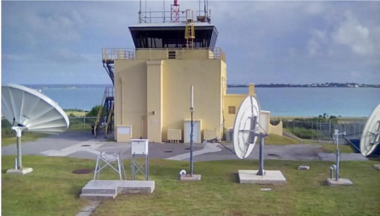
Air Traffic Control Tower, L.F. Wade International Airport looking south from BWS Ops Centre (Met enclosure in foreground) © Stephen Meloche, summer 2016
